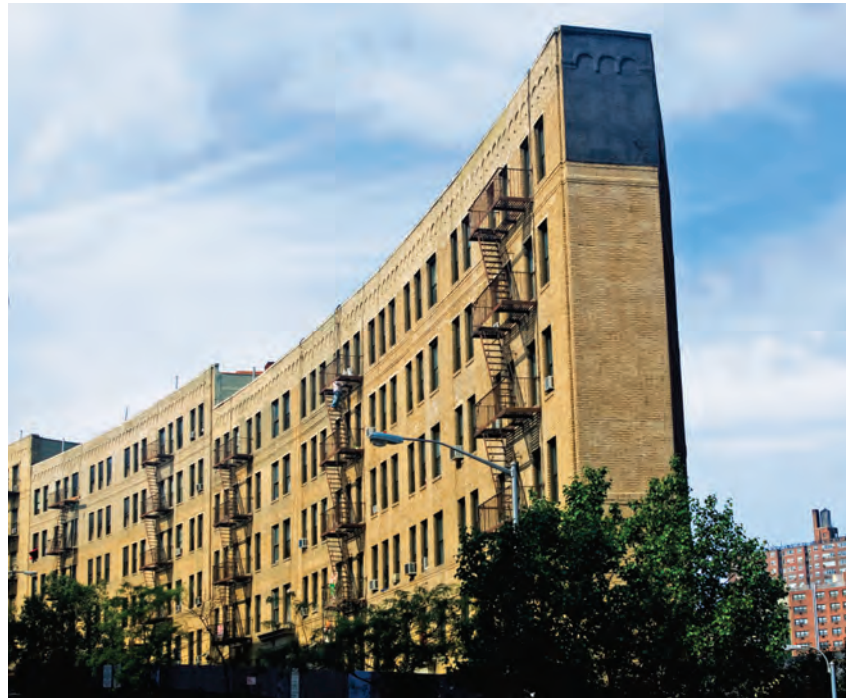
New energy efficient boilers, lighting and windows were installed in this 83 unit residential building located in Manhattan's Washington Heights neighborhood as part of a recent CPC-financed rehabilitation.
